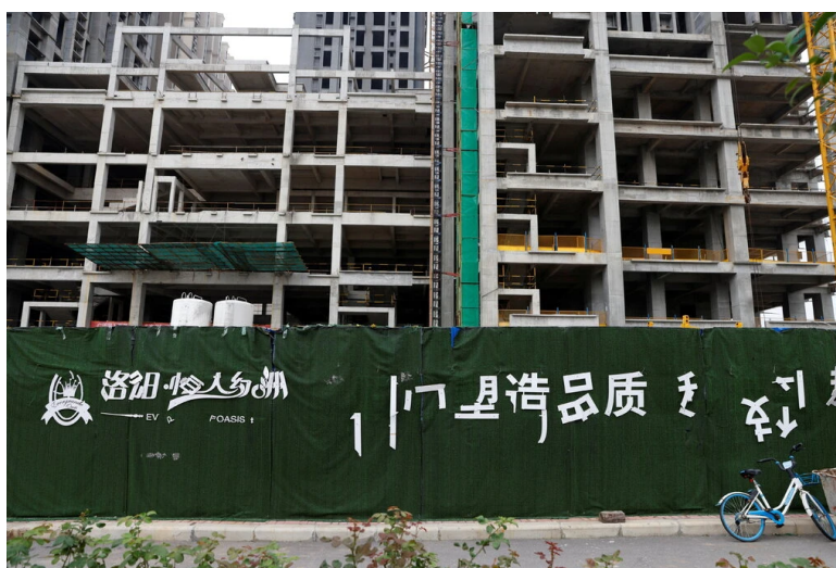
An unfinished Evergrande housing complex in Luoyang, China. Carlos Garcia Rawlins/Reuters
